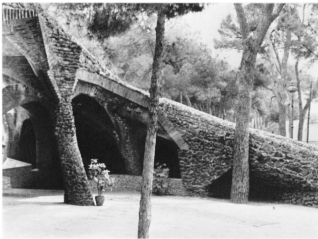
Fig. 9. Gaudí, Church at the Colonia Güell, Sta. Coloma de Cervelló. Porch of the crypt. The point of separation between column and arch (left) or wall and arch (right) is no longer certain (photo: author).
