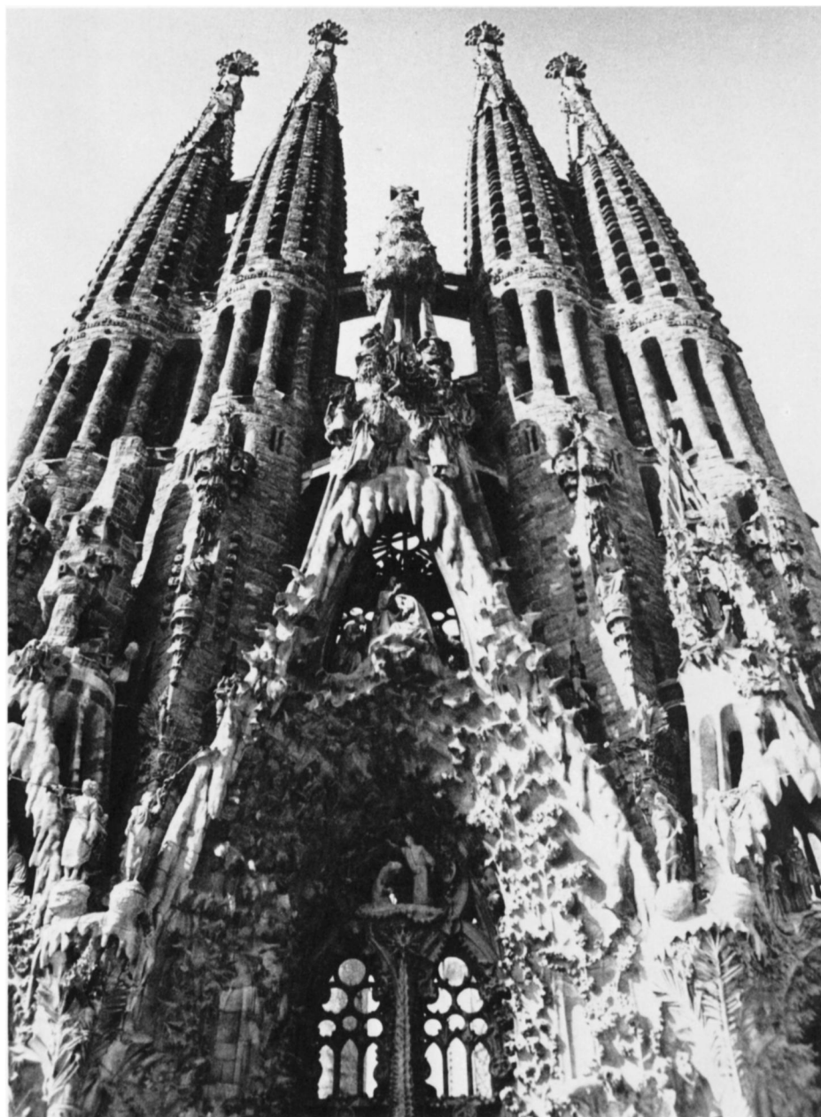
Fig. 13. Gaudí, Church of the Sagrada Família, Barcelona. Façade of the Nativity. The towers are simple paraboloids, recalling the frank geometry of mediaeval Catalan towers. The upper ends of the angled projections are masked by balconies. At the bottom is part of the central tympanum which Gaudí intended to fill with glass (photo: author).
